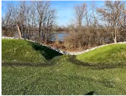
Fly Ash Pond Cap – Outlet 3 and embankment (facing north and south)
